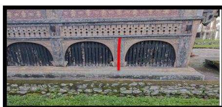
Figure 5. Under area of Rumah Gadang
