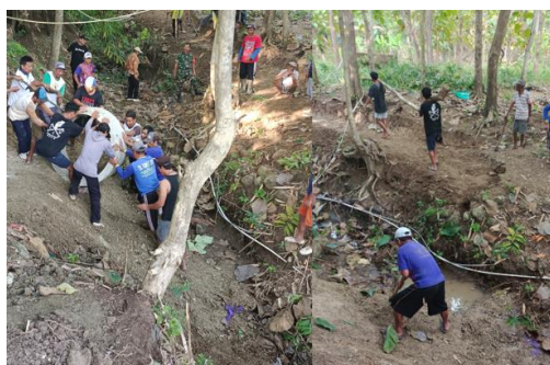
Figure 3. Residents installing irrigation for public baths (author's collection)
