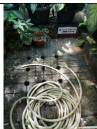
Figure 2. Infiltration wells (personal documentation)
