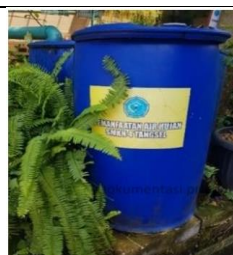
Figure 3. Rainwater catchment (personal documentation)
